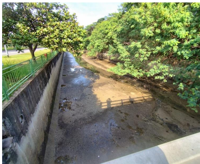
FIGURE 7-4: PUB DRAINAGE CANAL (ABOVE) AND OUTLET TO THE SEA (BELOW)
